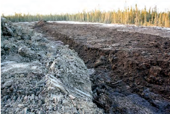
A. Clay to be removed (left side) and the completed clay peat inversion using the multi-step technique (right side).
