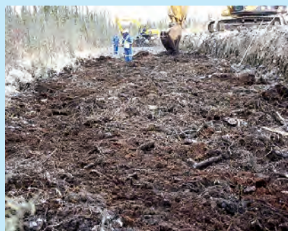
Figure 3. Left: The peat surface after clay removal waiting for fluffing. Right: The peat surface following fluffing.
