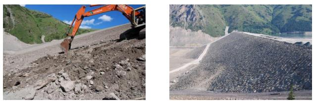
Photograph 1 (left) and 2 (right). Rough and loose surface configurations can be made using an excavator on slopes up to 2:1 or 26°. Large areas can be treated for a cost of about \$700/ha.
