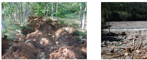
Photograph 3 (left) and 4 (right). Forest access roads and other small areas can be treated using the rough and loose technique (left) as well as areas with coarse substrates (right) such as this old dam site with alluvial boulders, cobbles and gravels.
